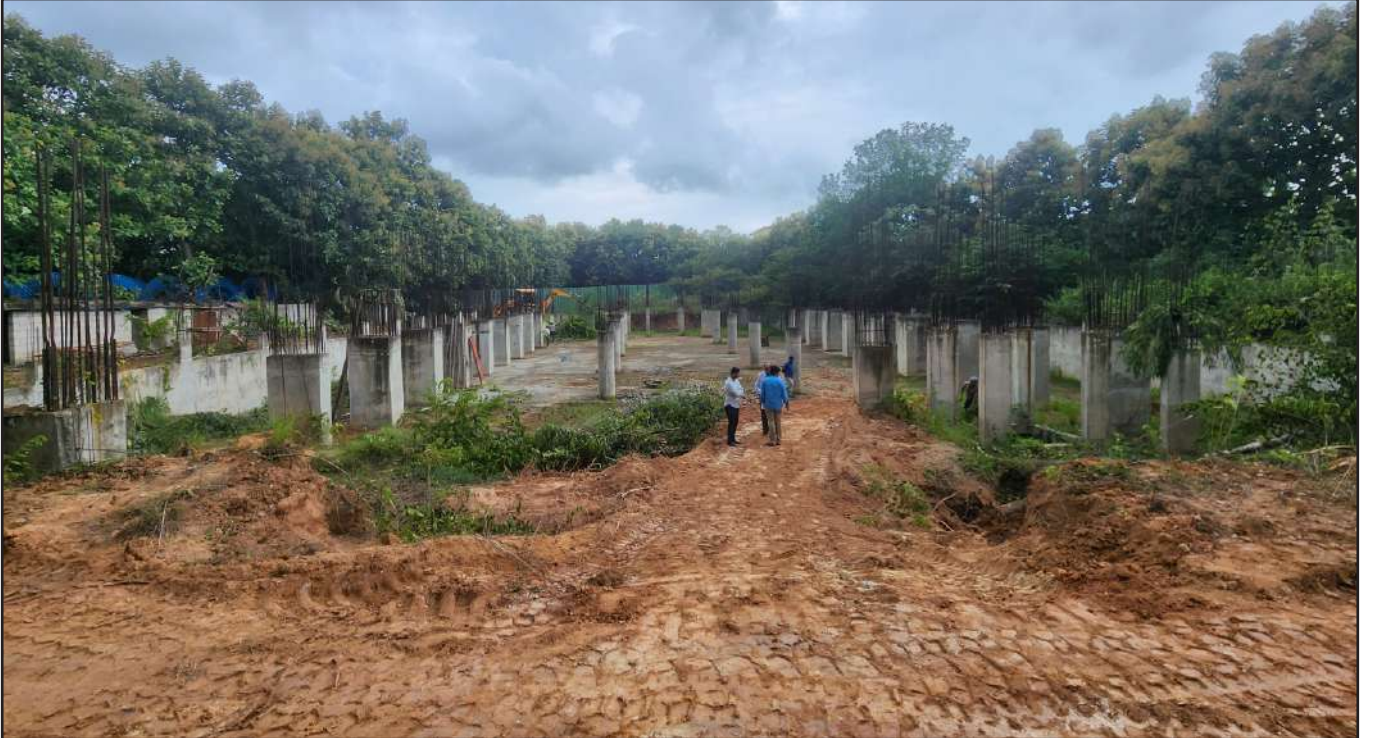
Photo of the Foundation works of Peenya Building which was stopped
